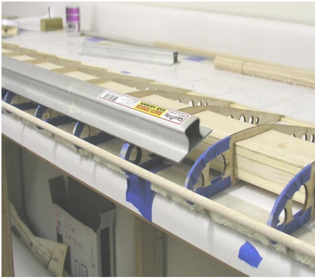
Tape rib noses, sand leading edge to shape
