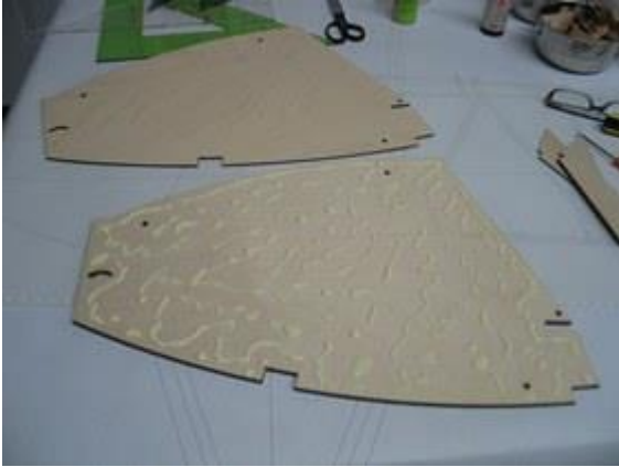
Glue forward plywood parts
