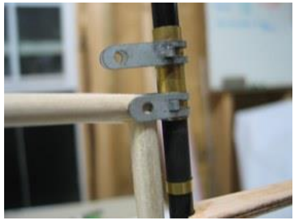
Drill 7/64 diameter hinge hole
