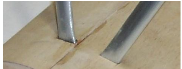
Plywood sheeting and strut #307, #308
