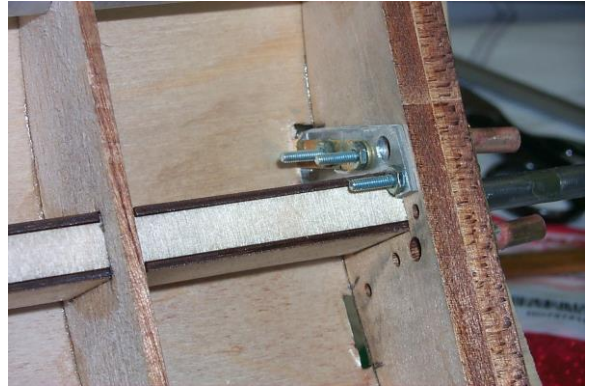
Cut slots in plywood covering for struts
