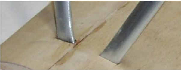
Plywood sheeting and strut #307, #308
