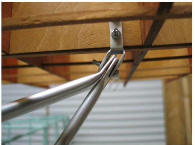
Another view of struts and fitting
